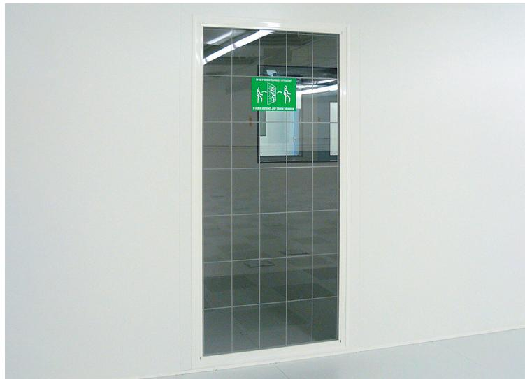
The Emergency Exit Break Barriers are the easiest and cleanest system to close the exits in Cleanrooms, requiring a minimum amount of space and opening radius when compared with traditional hinged doors: furthermore, the totally transparent surface permits continuous inspection of the emergency exits by the staff.
